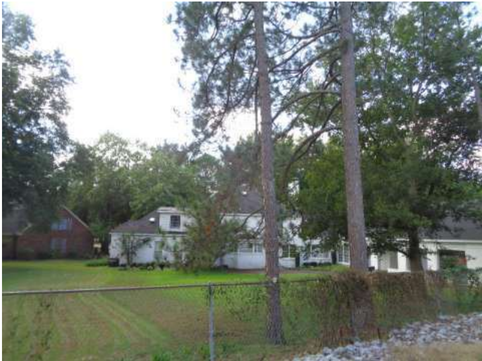
View to the South (Hines Street Site)
