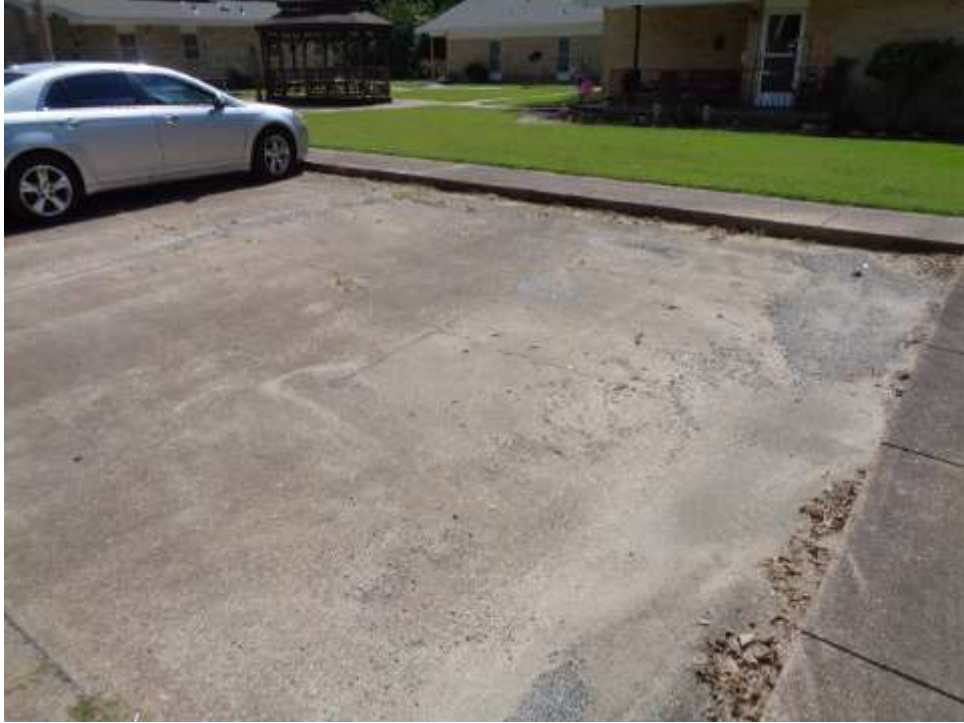
View of Parking
